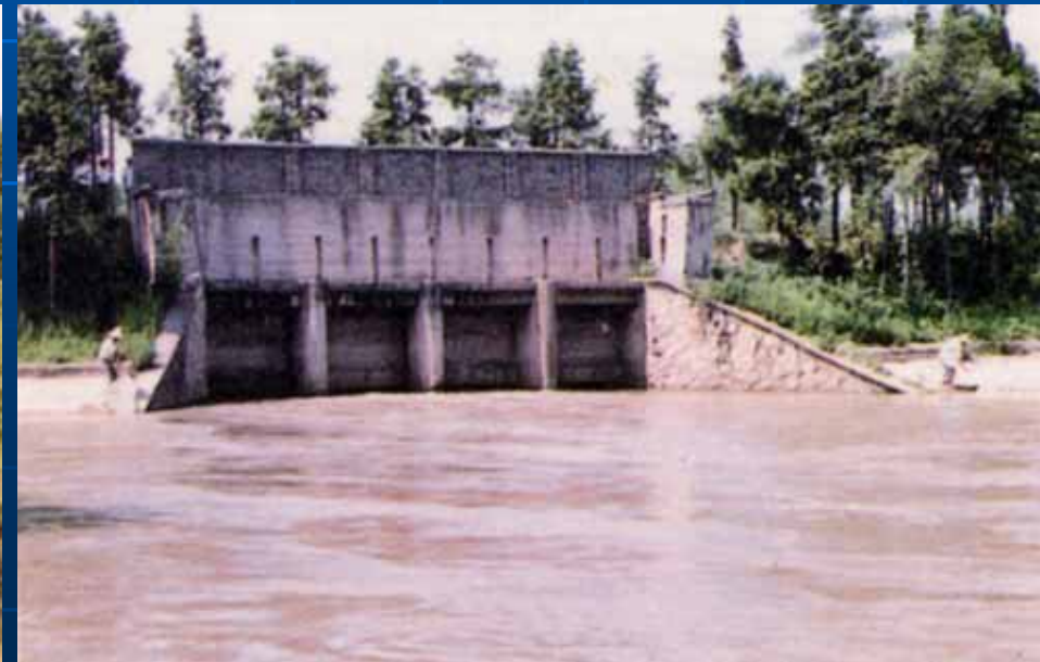
Floodgate of four hole
